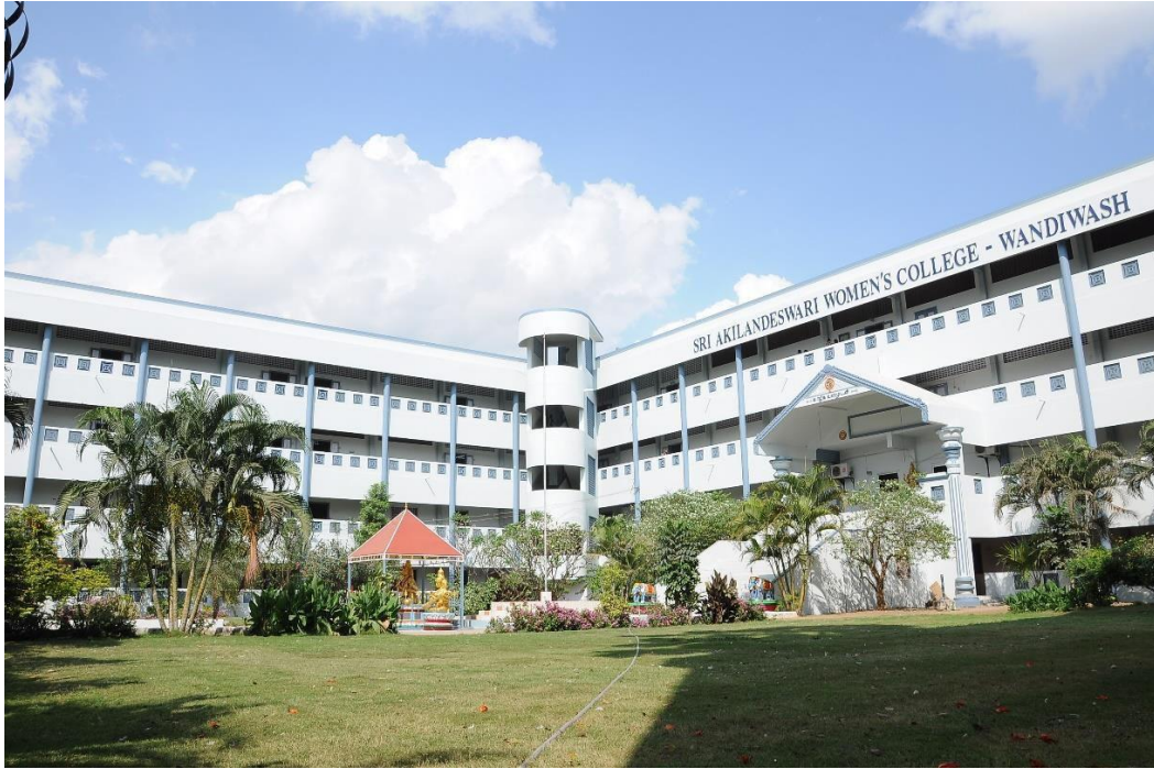
Fig. 4. View of the Academic Buildings
